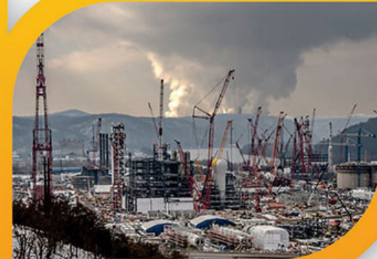
PLANT CIVIL WORK AND TOWNSHIP CONSTRUCTION
